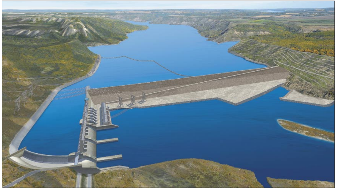
A rendering of BC Hydro's proposed Site C Clean Energy Project. Construction of the $7.9-billion hydroelectric dam and generating station would create 10,000 person-years of construction employment. Supplied photo
